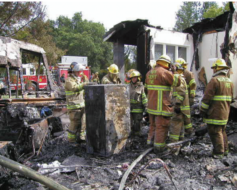
When keeping vital records on-site, it is recommended that education institutions store them in a fire-resistant file cabinet or vault that has been tested and rated by Underwriters Laboratories.
